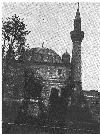
This mosque in Silistra, Bulgaria, is now closed. The notice on the boarded-up doors says "Cultural monument under repair". We report the situation of Turkish Muslims in Bulgaria in the Chronicle item on pp. 209-12.
