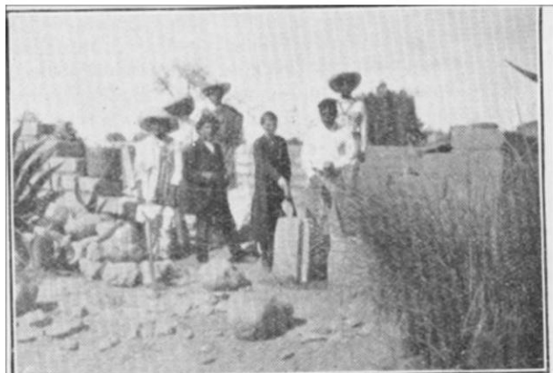
Mrs. Thomas laying a stone for the new Church
