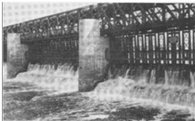
Sluice Gates and Bridge over the Red River, near Winnipeg.
