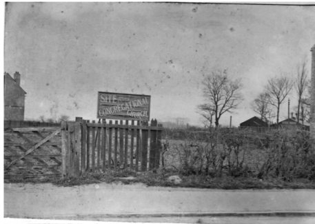
Site for proposed new building on Grovehill Road
